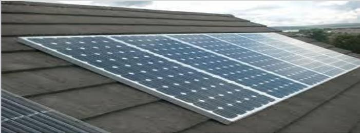
**Photovoltaic Solar Panels** - A typical silicon PV cell is a thin wafer consisting of phosphorous doped (N-type) silicon on top of a thicker layer of boron-doped (P-type) silicon. An electric field is created near the top surface of the cell where these two materials are in contact (the P-N junction). When sun light strikes the surface of PV cell, this electrical field results in a flow of current when the cell is connected to an electrical load.
